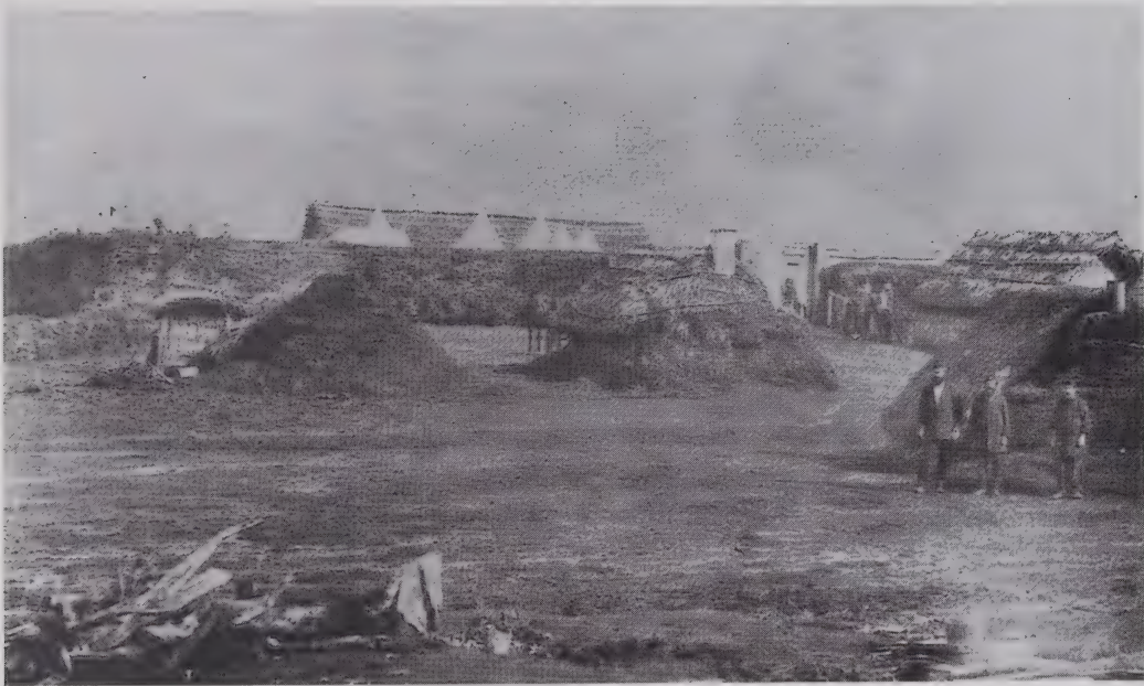
Fig. 12. St Andrew's Redoubt. The camera has been set up beyond the small shed in the left foreground of Figure 11, to show the redoubt with tents, signal mast and large raupo-roofed huts within. A causeway with handrail leads to the gateway. In the foreground cooking is going on over an open fire. (Volume 2, Nicholl Albums, Alexander Turnbull Library, Wellington).
